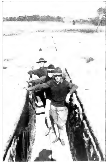
Section of trenches at Camp Hancock, Augusta, Ga.
